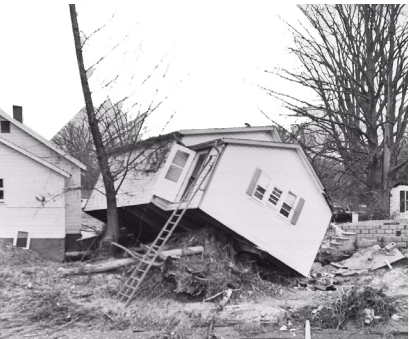
DESTRUCTION CAUSED BY HURRICANE HAZEL
