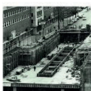
Construction station Berri-de-Montigny, 1963
