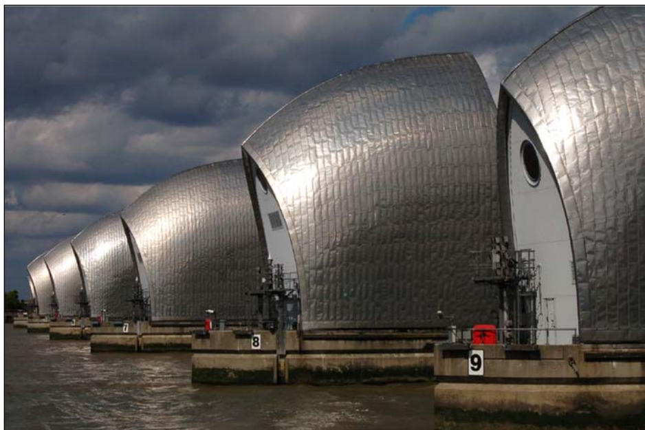
The Thames Barrier is operated by the UK Environment Agency and protects London from major storm surge events. The National Oceanography Centre work closely with the Environment Agency to help define the threshold levels at which the barrier should be closed.
