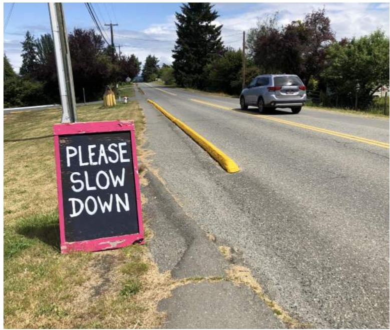
Asphalt Curb Sidewalk
