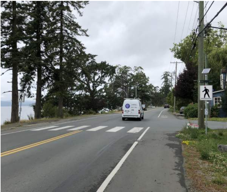
Zebra Crosswalk with RRFB
