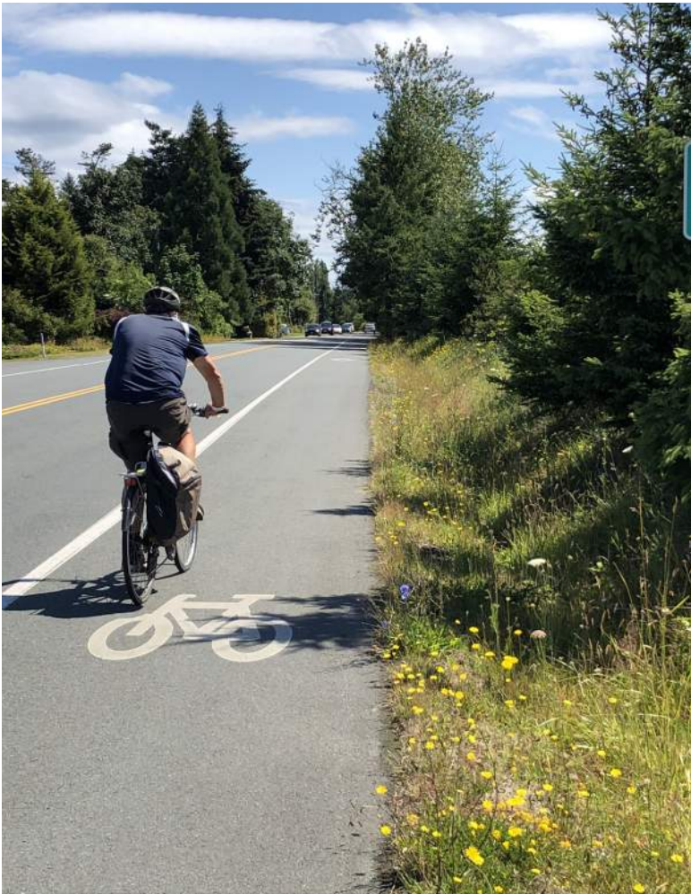
Painted Bicycle Lane
