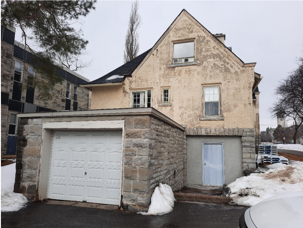
Rear Elevation (South) showing modern flat roof garage addition
