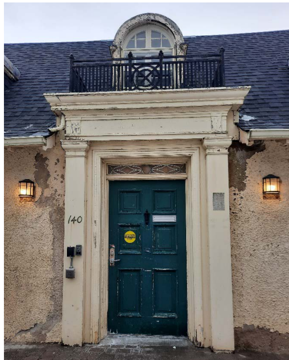
Front Entrance (North) – Six-panel wood door with decorative leaded glass transom with classically influenced wood surround and small balcony with ornamental metal rail above
