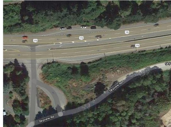
Island Highway and Skyview/Hillview Road
