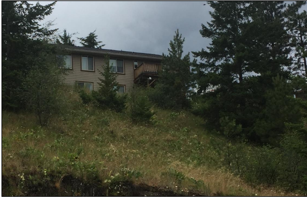
FIGURE 13 Combustible decks need to be assessed for ember accumulation features, such as flammable patio furniture and other combustible items stored on or underneath. Decks that extend out over a slope require careful assessment of the fuel conditions downslope. A deck overhang can concentrate heat from a fire coming up the slope and lead to an increased probability of ignition.
