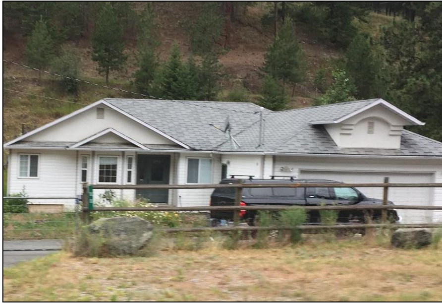
FIGURE 17 A rated roofing system, such as this composite shingle roof, provides fire-resistance to embers. Any modern roofing system that has a fire-resistance rating can provide this protection.
