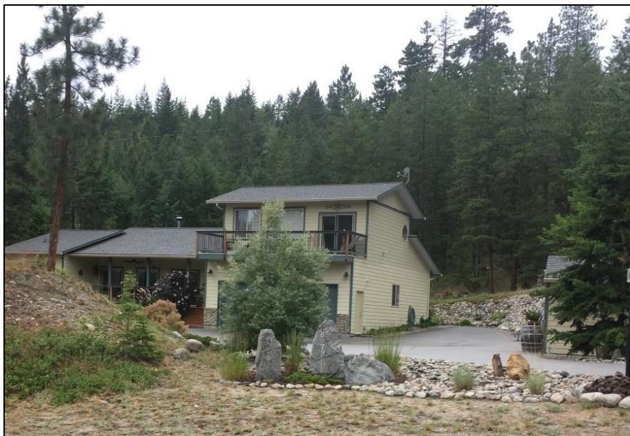
FIGURE 18 The combination of paved or gravel surfaces, rock ground cover, green lawn and rated roof all contribute to the fire resilience of this home.
