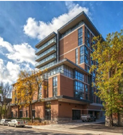
The One32 Berkeley building developed by Concert Properties is a certified TGS Tier 2 building.
